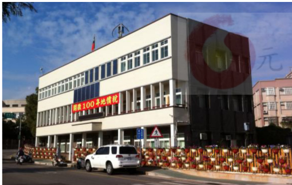
圖 2.8 完工後立面太陽能建築一體 (BIPV) 複層式外牆的模式 Figure 2.8 Building-integrated photovoltaics (BIPV) were installed, with a composite wall design.
